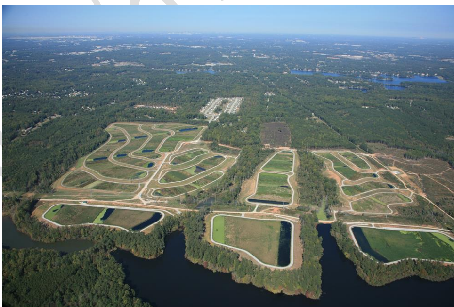
Figura 37 – Caso- North Texas Municipal Water District's East Fork Water Reuse Project
